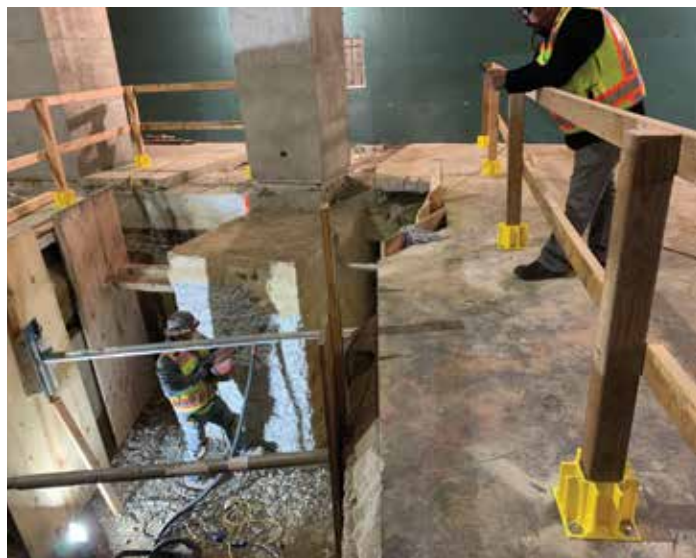
Scarification of existing foundation concrete.
