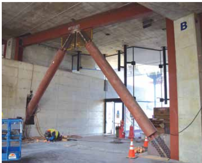
Installing braced frames adjacent to existing concrete.
