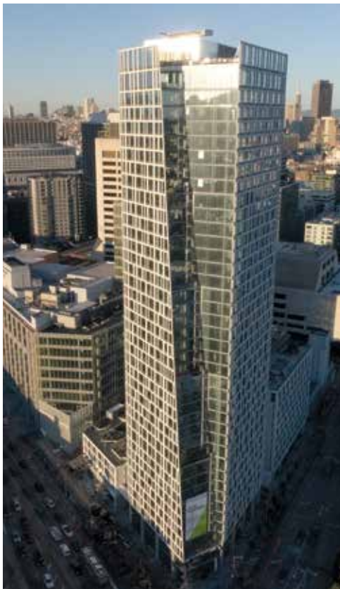
Stepped-back waterfall balconies created unique framing challenges at the Mission and Van Ness corner.
