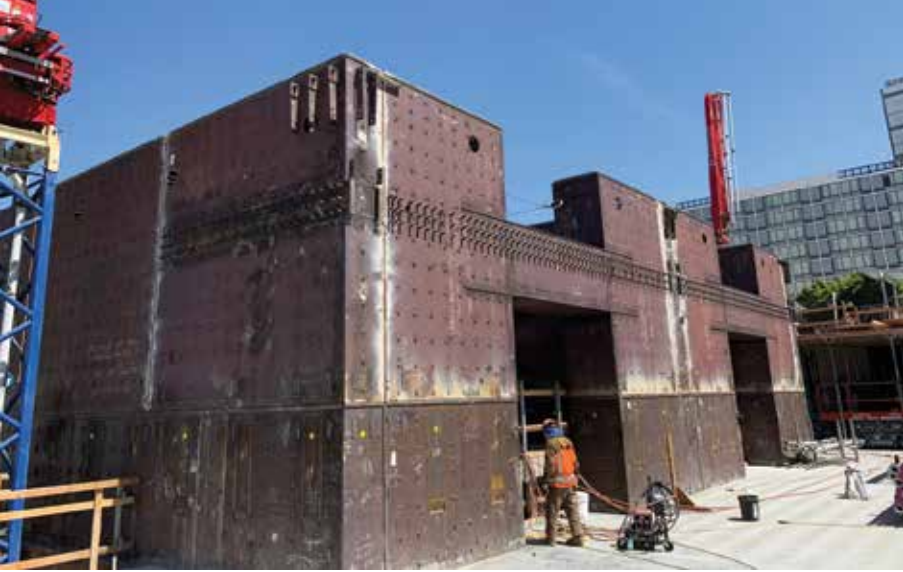
Figure 3. Prefabricated empty steel module of coupled C-PSW/CF for 200 Park Avenue high-rise.
