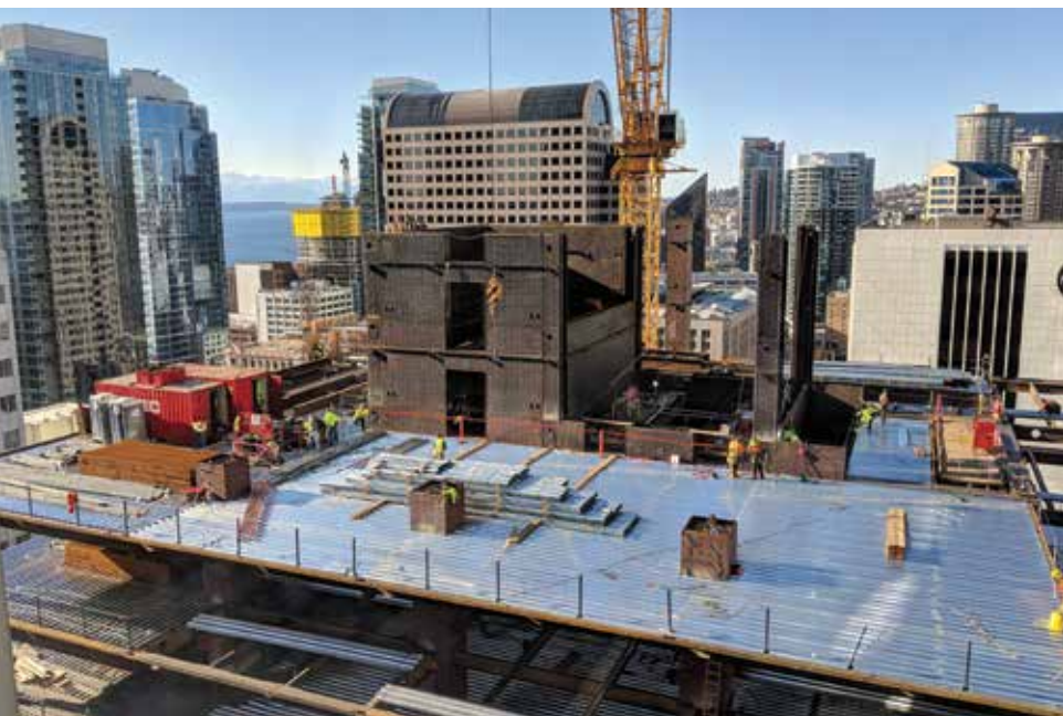
Figure 2. Construction of Rainier Square Tower in Seattle.
