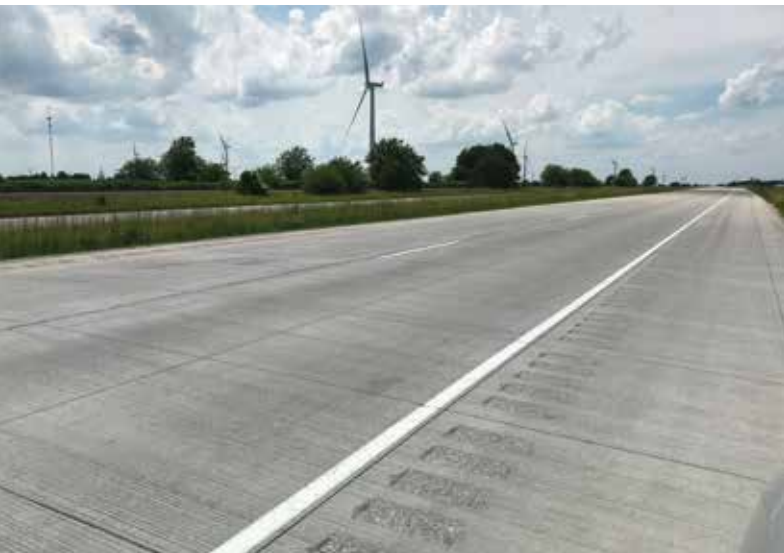
Concrete overlay with macrofibers in Indiana.
