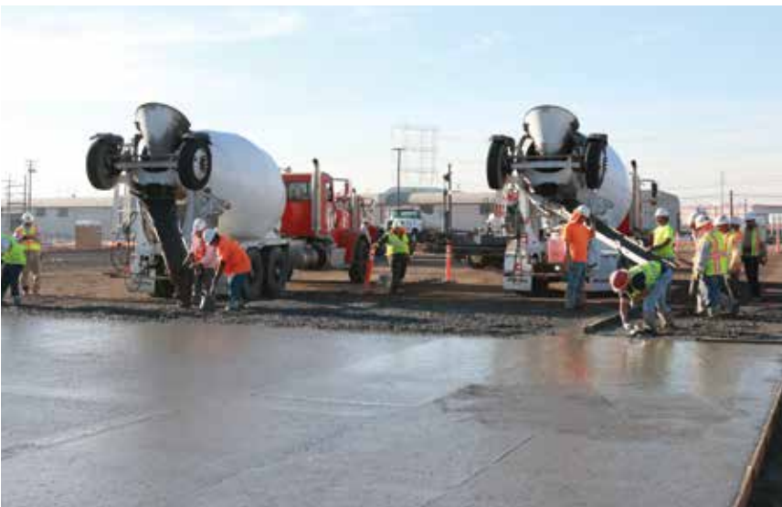
Warehouse construction in Arizona using synthetic macrofibers.
