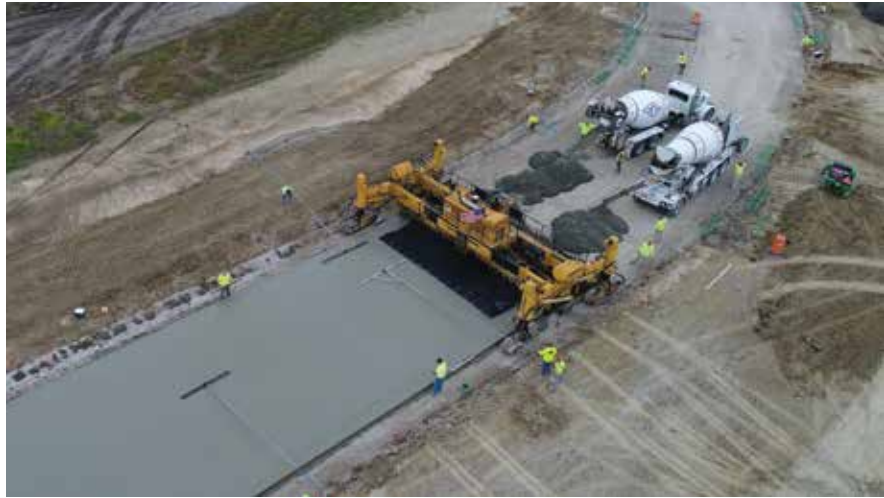
Full-depth concrete paving with macrofibers in Ohio.
