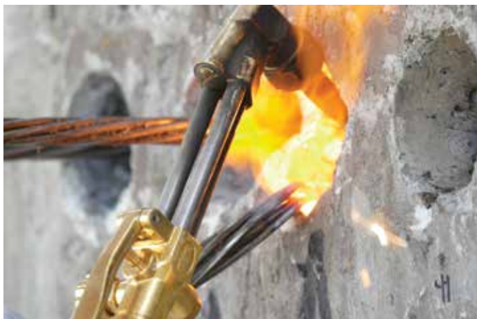
Figure 2. Cutting a tendon tail using an oxyacetylene torch.
