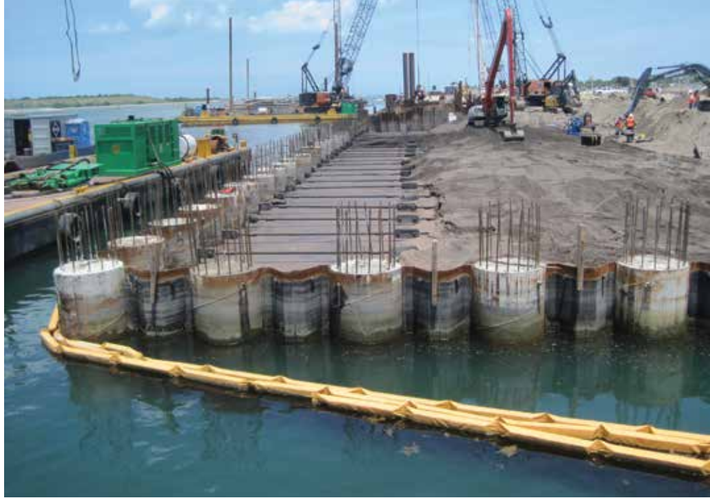
Lightweight fill being placed behind the combi-wall. Courtesy of Gary Ledford.
