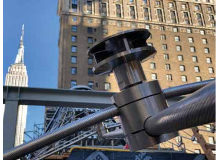
Construction of glass clamp at cable intersections.
