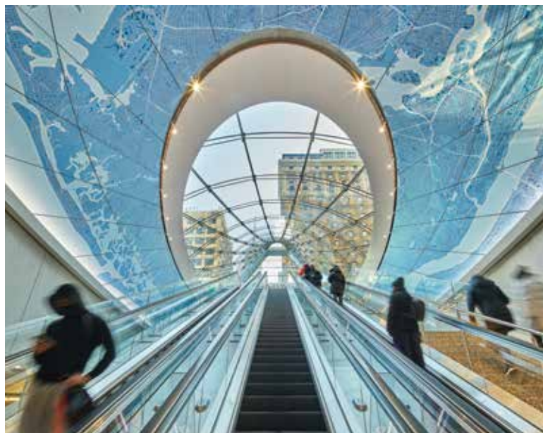
The east end gateway allows direct access to the concourse and brings natural light into the space for the first time.
