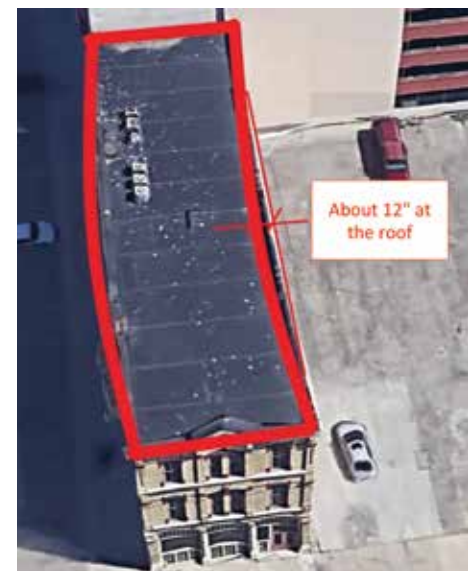
Figure 3. Exaggerated view of building displacement (left) and an aerial view from Google Earth (right) before renovation. The decorative street façade faces south.
