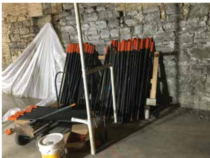
Figure 5. 1½-inch threaded steel bars for micropiles, staged in the basement.
