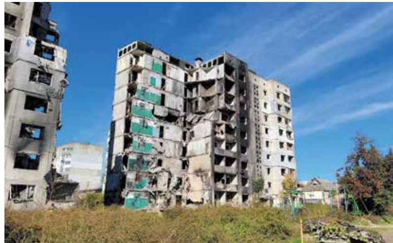
Kyiv apartment building devastated by deadly shell.
