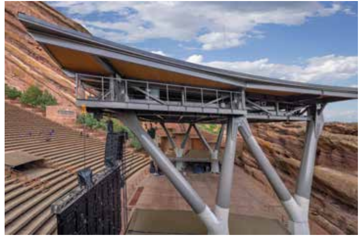
Side view of roof structure. Courtesy of Frank Ooms.
