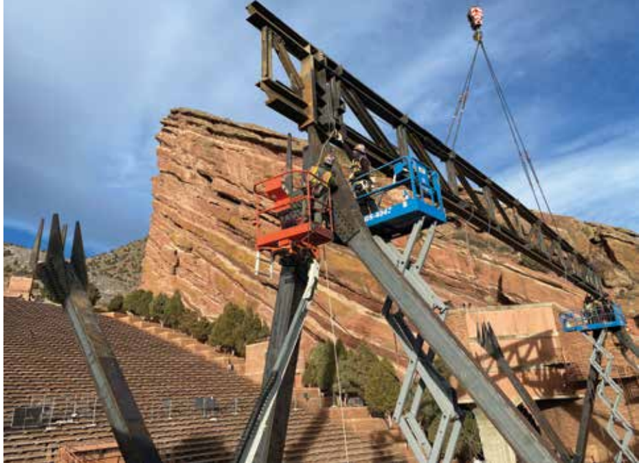
Figure 5. Center primary truss erection on "W" columns. Courtesy of GH Phipps.
