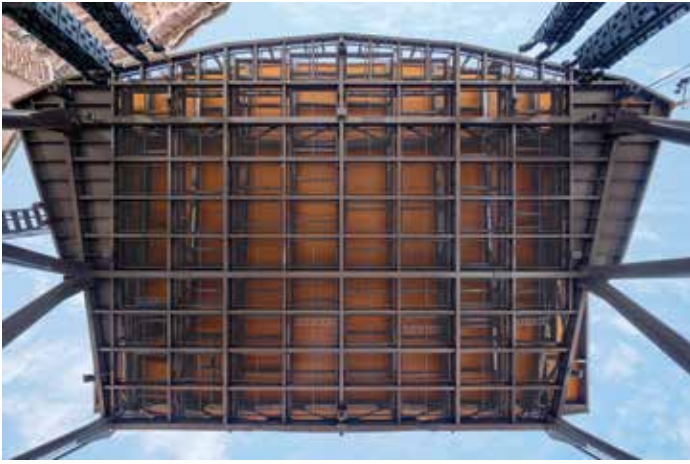
Underside of roof structure from stage. Courtesy of Frank Ooms.
