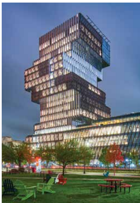
Center for Computing & Data Sciences nearing completion. Courtesy of John Cannon Photography.
