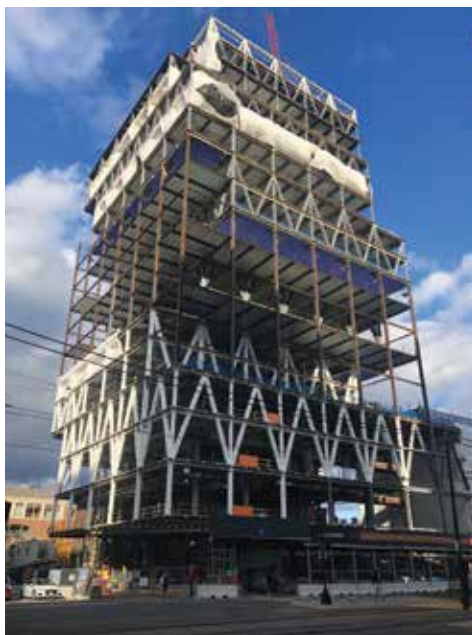
Steel framing with temporary shoring (left); Steel framing after shoring removal (right). Courtesy of John Cannon Photography.
