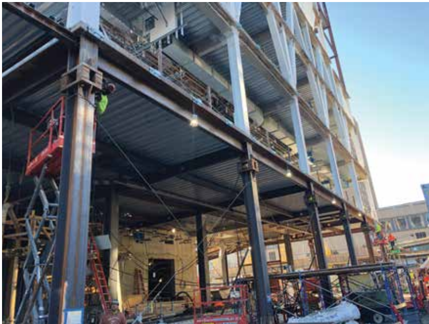
Temporary shoring at tower base during shoring unloading.
