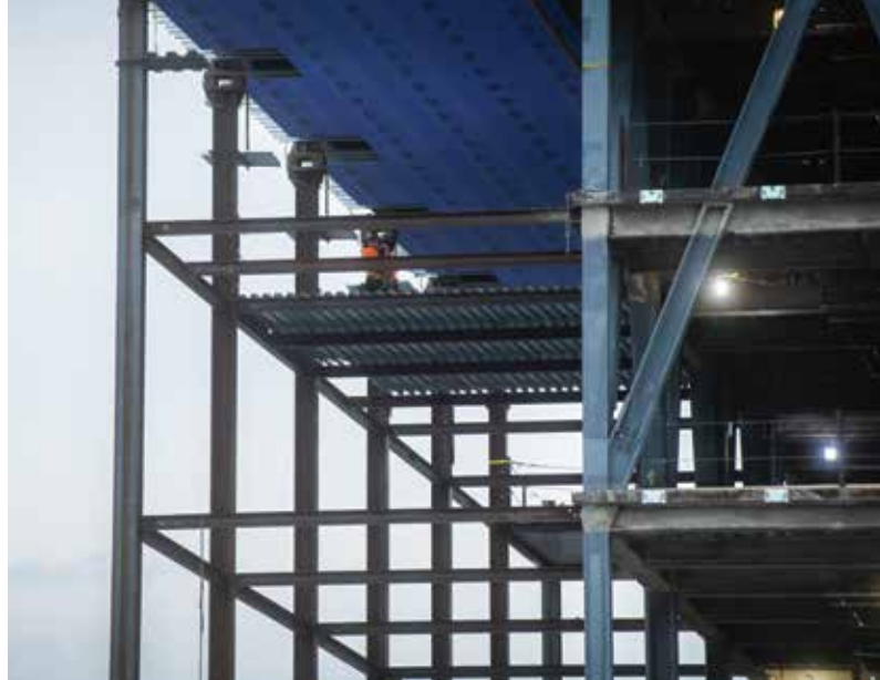
Temporary shoring. Courtesy of Cydney Scott/Boston University Photography.
