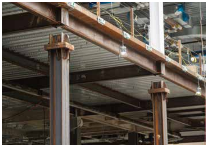
Jack box after removal.
