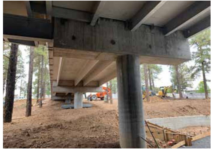
Figure 6. Bridge connected pedestrians to nature while reducing cost and preserving trees.
