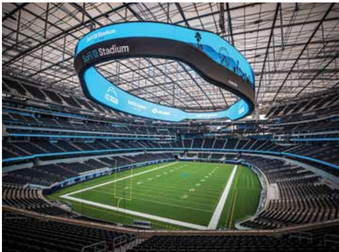
SoFi Stadium in Inglewood, California, used a semitransparent membrane as the roofing material of choice due to the material's higher mechanical strength and thermal performance. Courtesy of SoFi Stadium and Hollywood Park.
