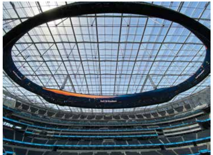
SoFi Stadium in Inglewood, California, has an ethylene tetrafluoroethylene roof to provide a protected and temperature-controlled environment. Courtesy of SoFi Stadium and Hollywood Park.
