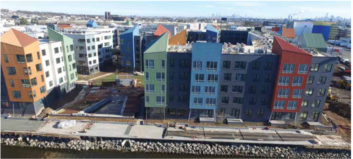
Example light gauge bearing wall podium with completed framing.
