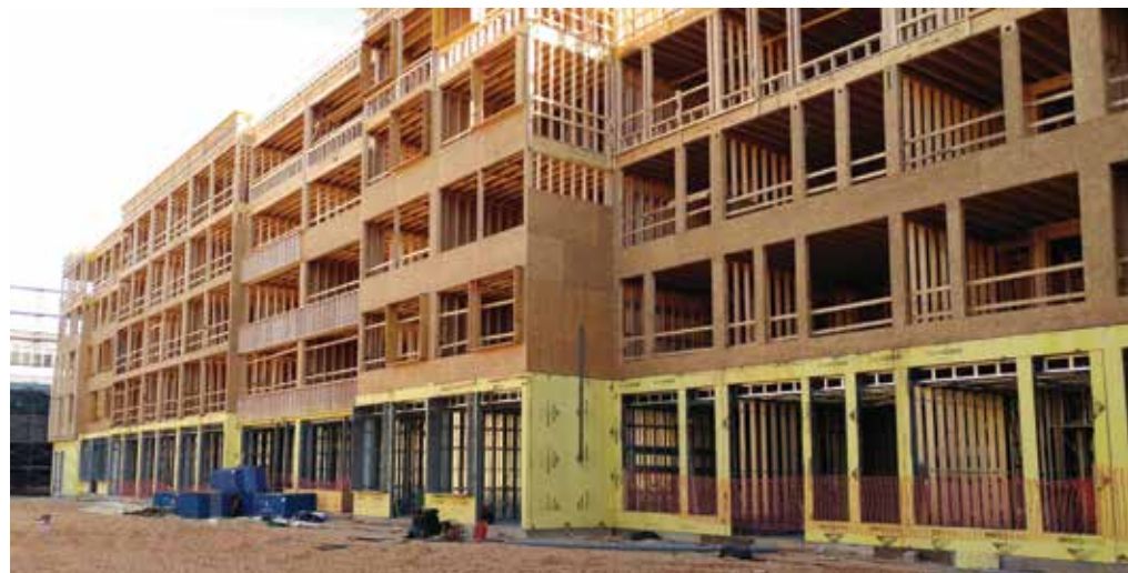
Stacking wood and light gauge CFS framing under construction.
