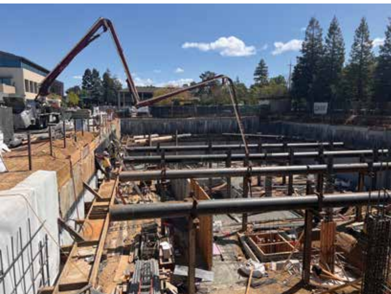
Figure 3. 1 st Street shoring.
