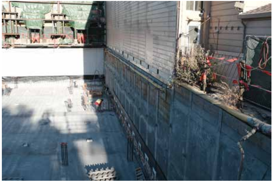
Figure 2. Underpinning.
