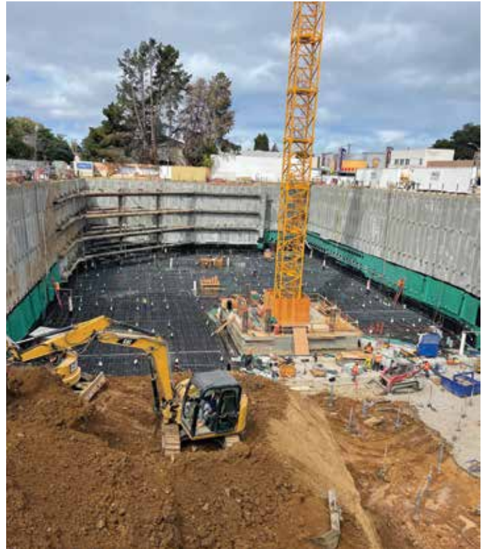
Figure 1. Baldwin temporary shoring.
