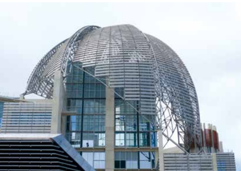
Galvanized AESS framing supports stainless steel cladding.
