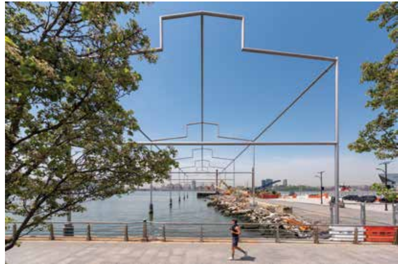
Permanent public art project with AESSS and custom cast stainless steel connections. Photography by Timothy Schenck, courtesy of the Whitney Museum.
