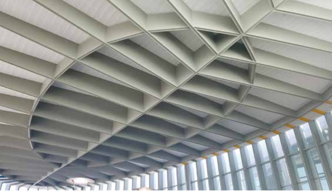
Expressive structural steel geometry.
