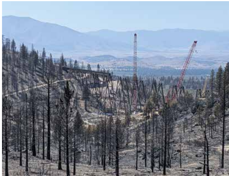
View of the span removal process working from Span 19 through Span 9.
