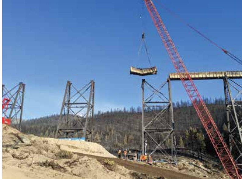
The removal of Span 10 looking east.
