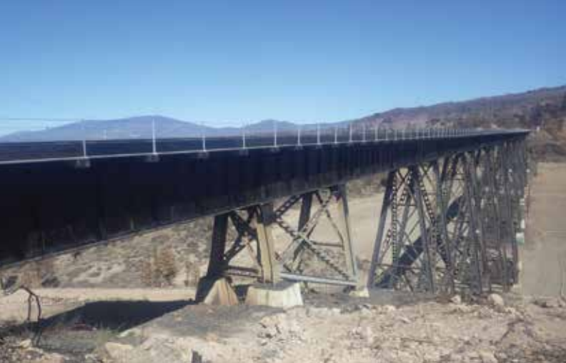
The completed, repaired bridge looking northwest from the south embankment.
