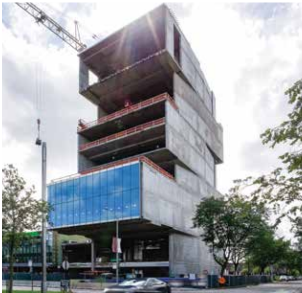
The tower's efficient form is derived from a box-like structure created by the unique stacking of slabs and cantilevered walls.
