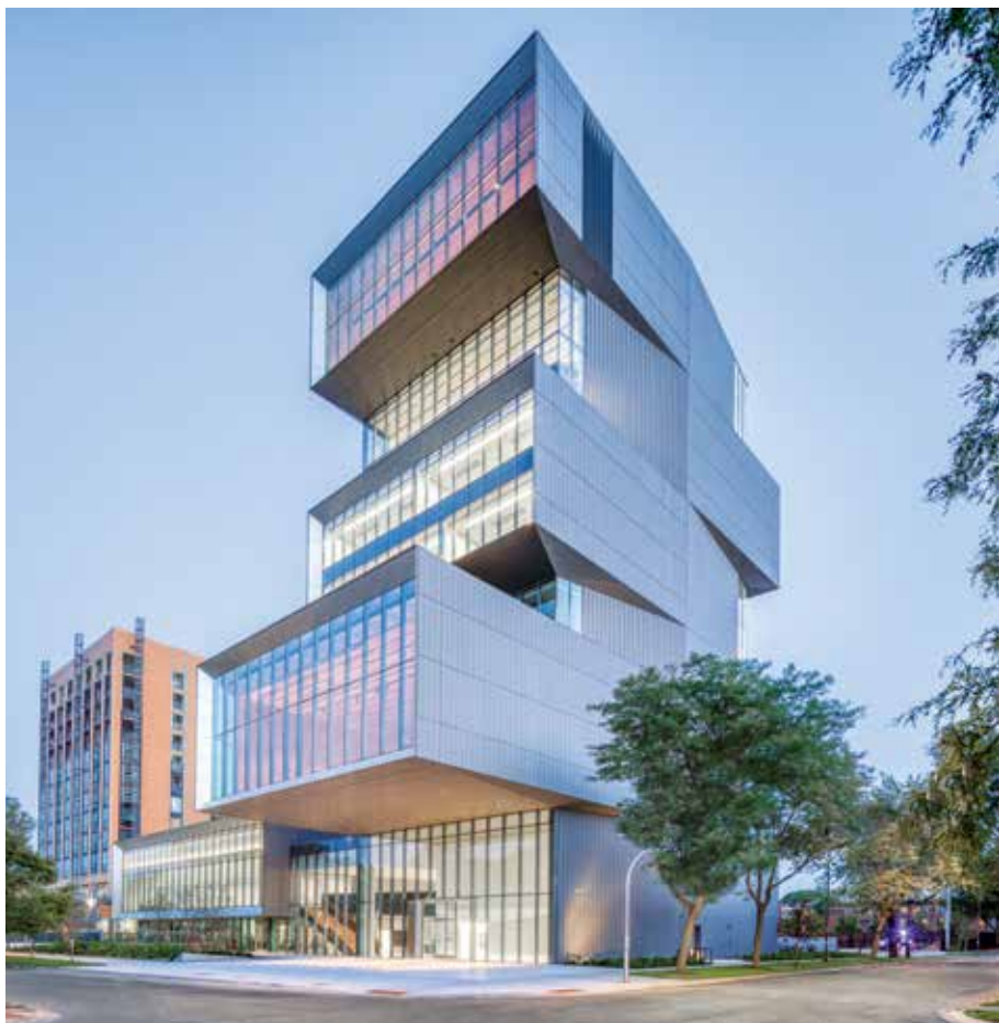
The staggered design of the tower features cantilevers of up to 40 feet. Courtesy of Brett Beyer.
