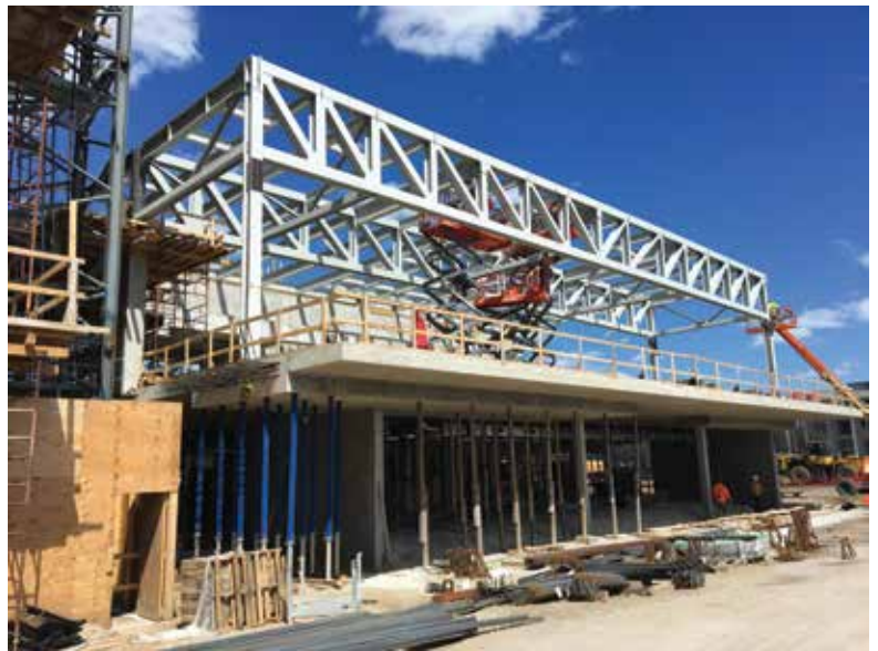
At the podium, a pair of steel roof trusses rest upon and are transferred by a system of cantilevered post-tensioned slabs and beams at Level 2.
