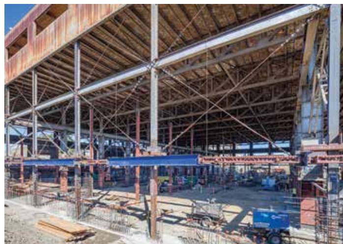
Figure 6. Shoring removed – the blue lifting beams and cable bracing remain.
