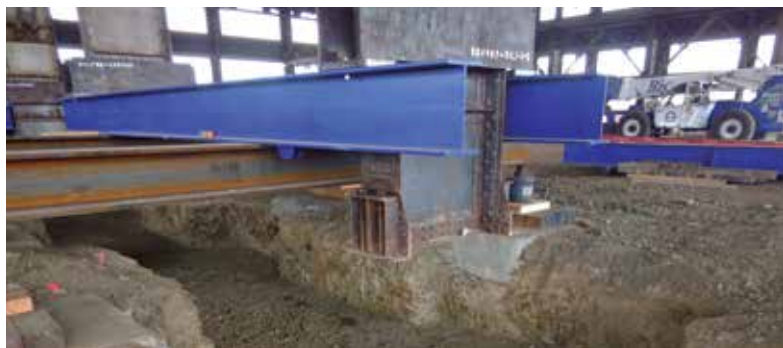
Figure 2. Initial lift with new foundations excavated.
