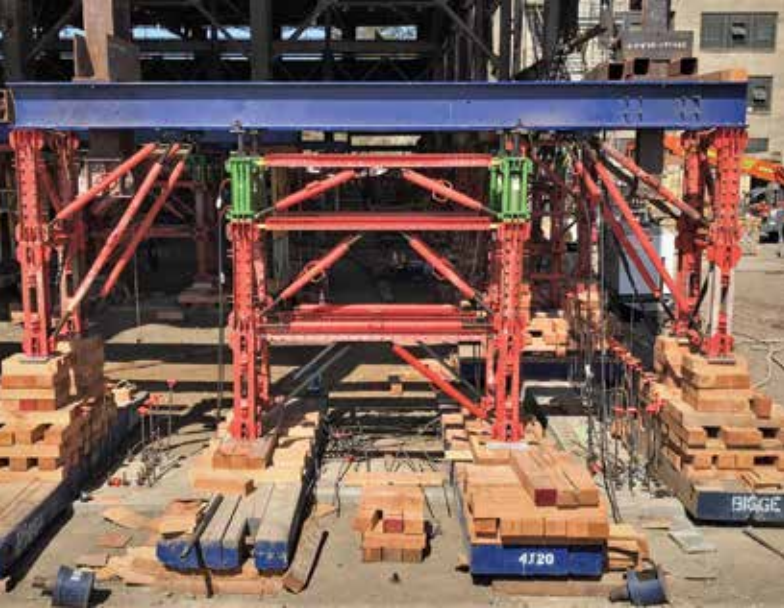
Figure 4. Full lift shoring.
