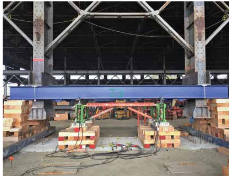
Figure 3. Partial lift shoring.
