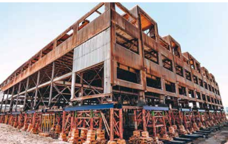
Figure 5. Building after the main lift.
