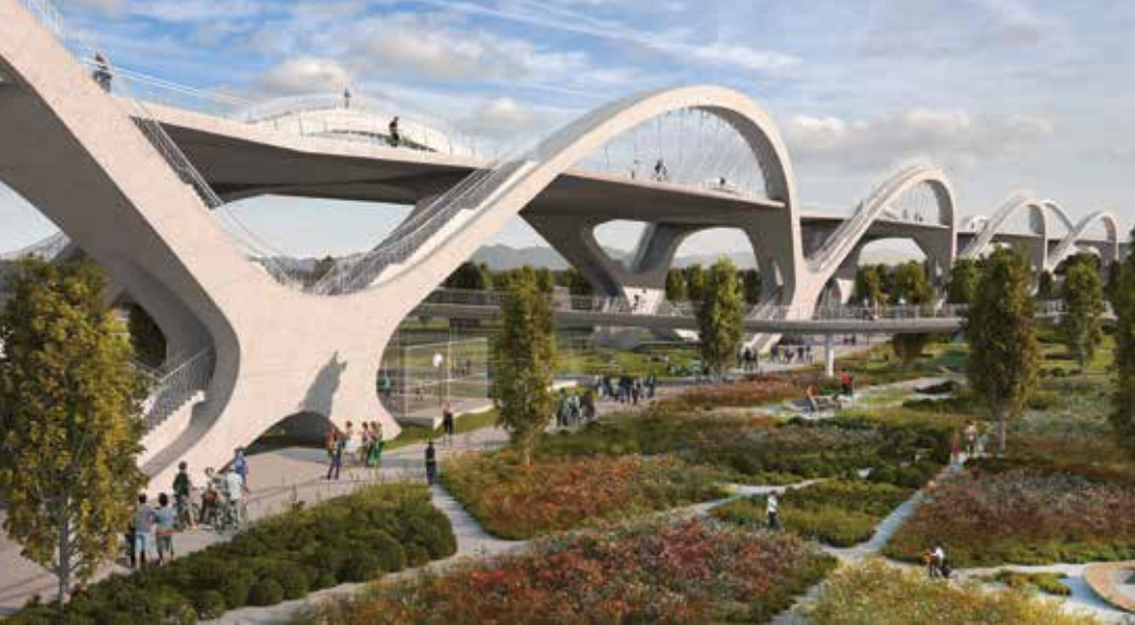
Rendering of X-pier substructure concept.
