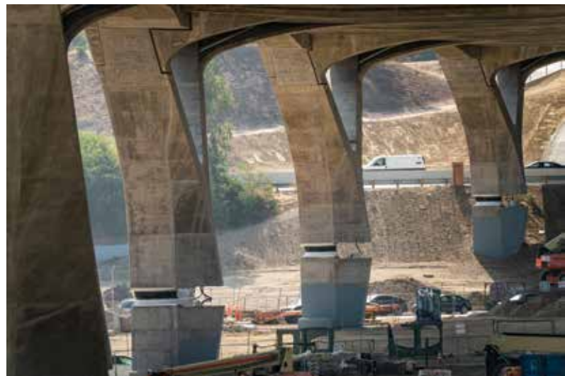
Isolation bearing placed within column height.
