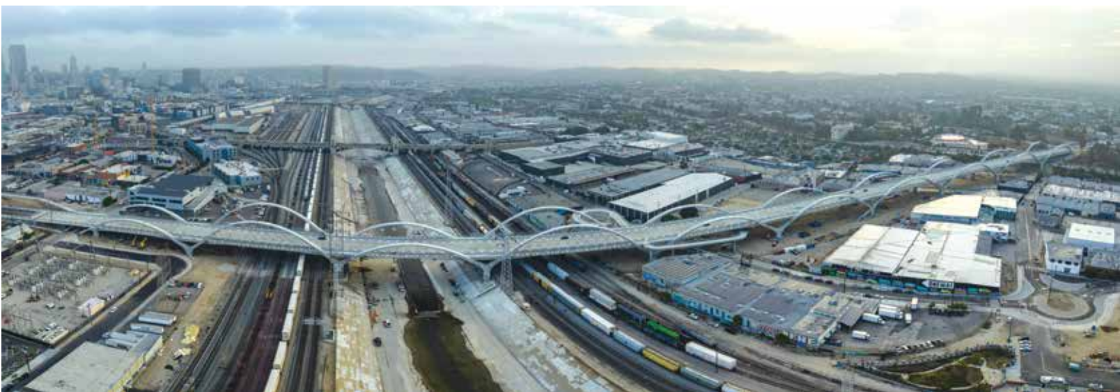
Aerial view of New Sixth Street Viaduct.
