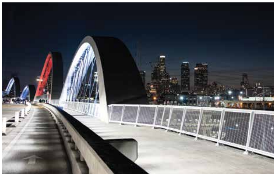
New Sixth Street Viaduct. Courtesy of JC Dick Photography.
