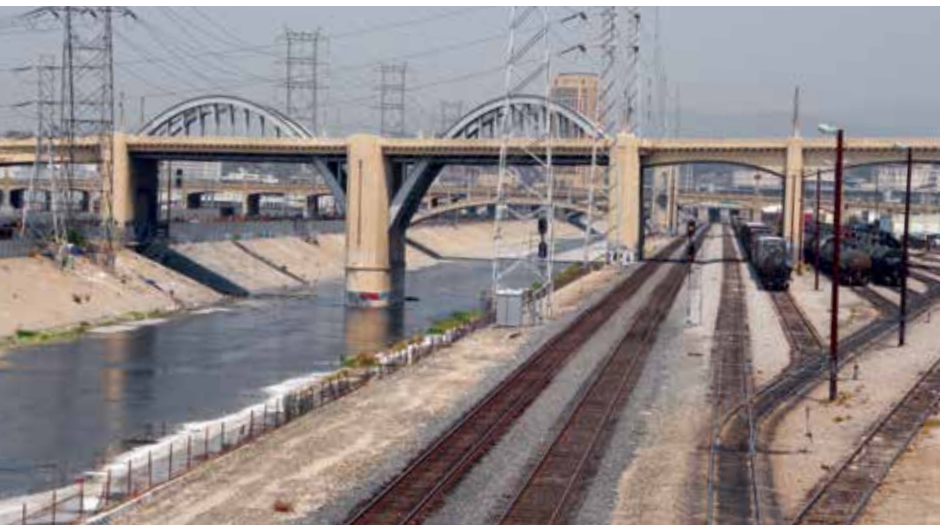
Original Sixth Street Viaduct. Courtesy of Gary Leonard.
