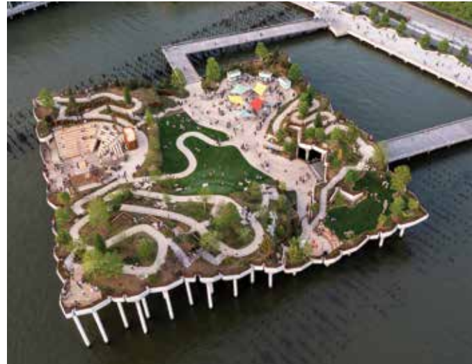
Arup was an Outstanding Award Winner for the Little Island Project in the 2021 Annual NCSEA Excellence in Structural Engineering Awards Program in the Category – Other Structures.
