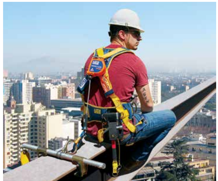
Figure 5. A sliding beam anchor anchored to structural steel.
