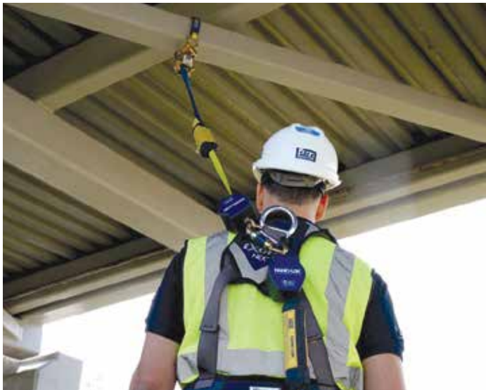
Figure 6. An SRL anchored to structural steel.
