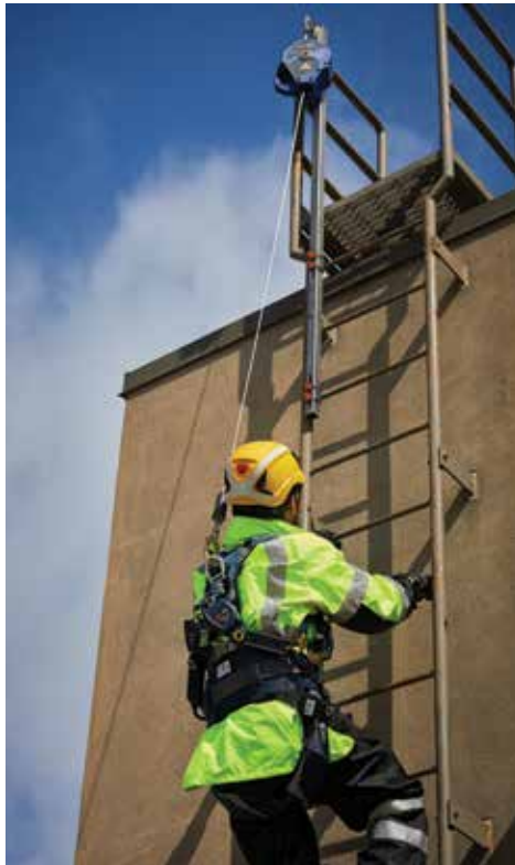
Figure 3. An SRL connected to a ladder anchor system anchored to a fixed ladder.
