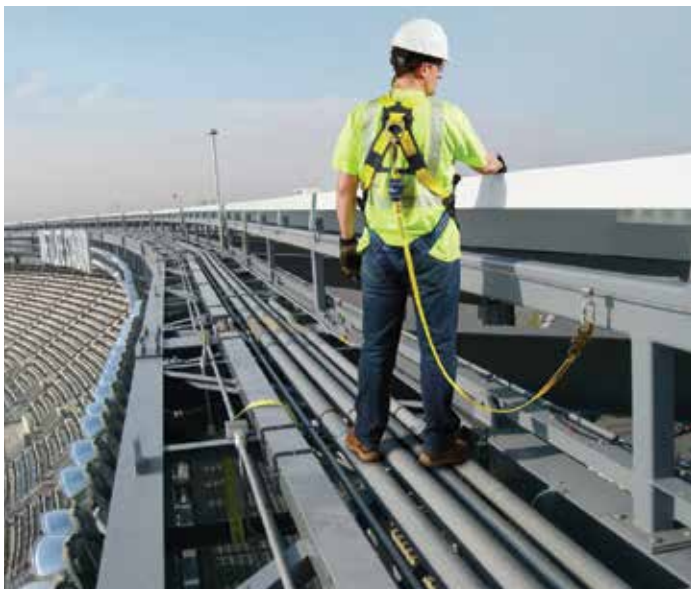
Figure 4. A lanyard anchored to an engineered permanent horizontal lifeline system.
