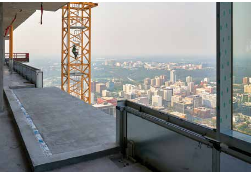
Figure 2. Concrete-to-concrete structural thermal breaks installed.
