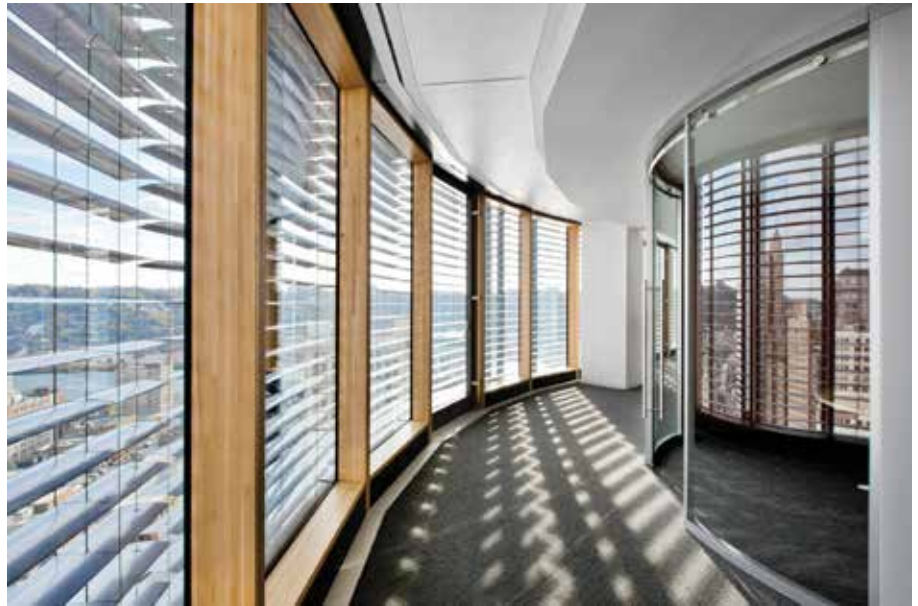
Figure 7. Interior and exterior curtain wall at PNC Plaza. Courtesy of Gensler.
