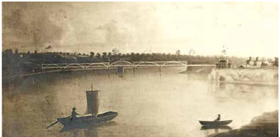
Western portion of the bridge with Rock Island on the right.
