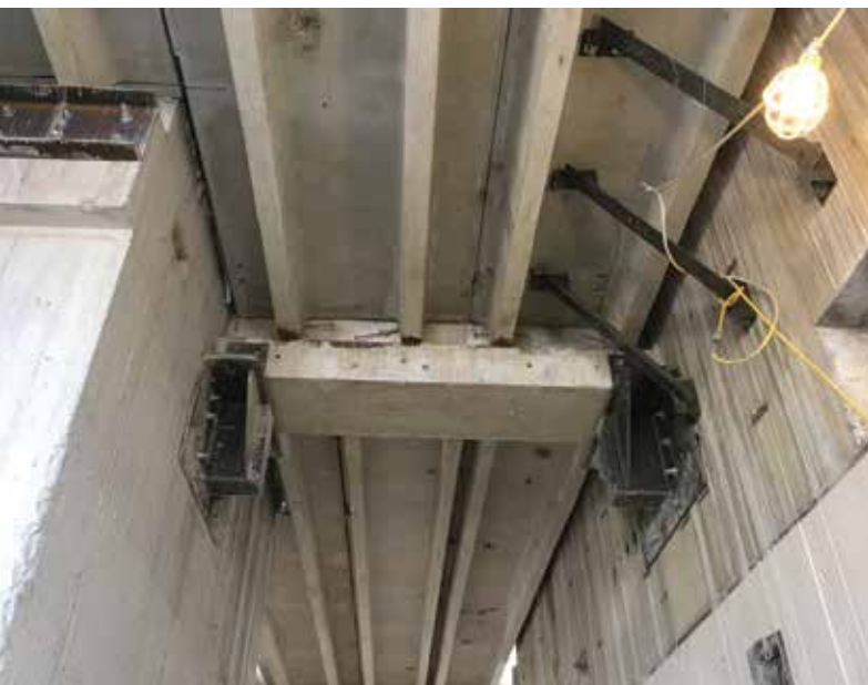
Figure 1. Concrete girders "released" from supporting wall with epoxied support brackets.
