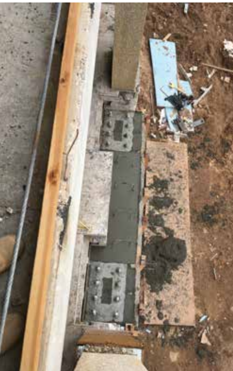
Figure 5. BRBF keyed into the existing foundation wall system.
