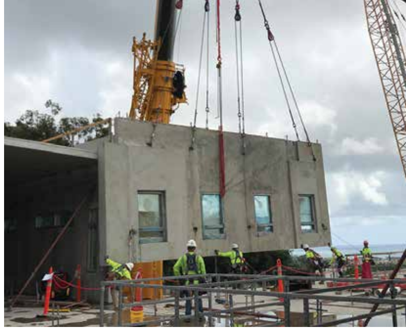
Figure 3. Installation of the precast wall panel with the cast windows.
