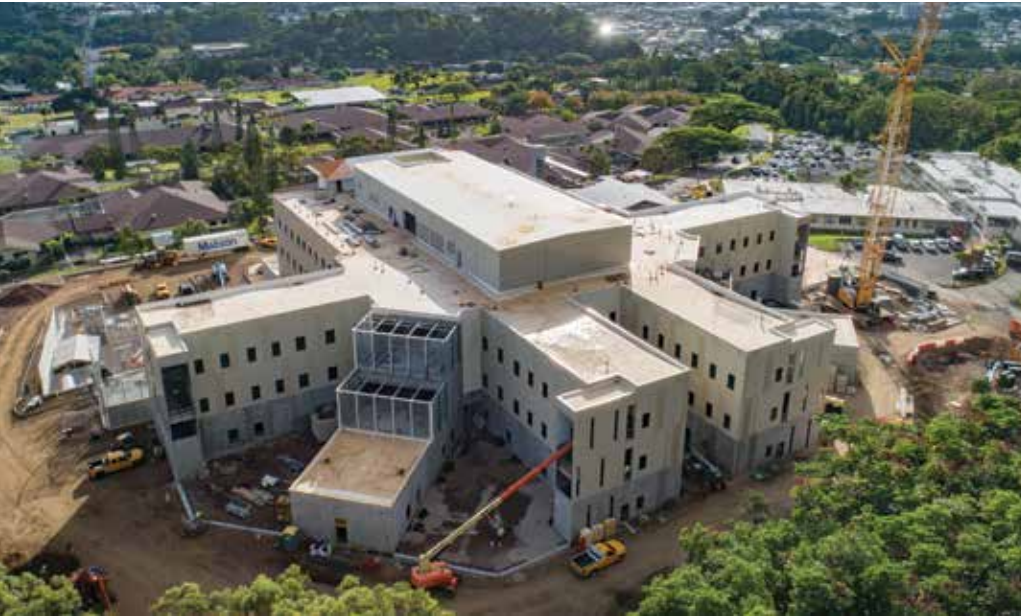
Figure 1. Construction of the new patient wings.
