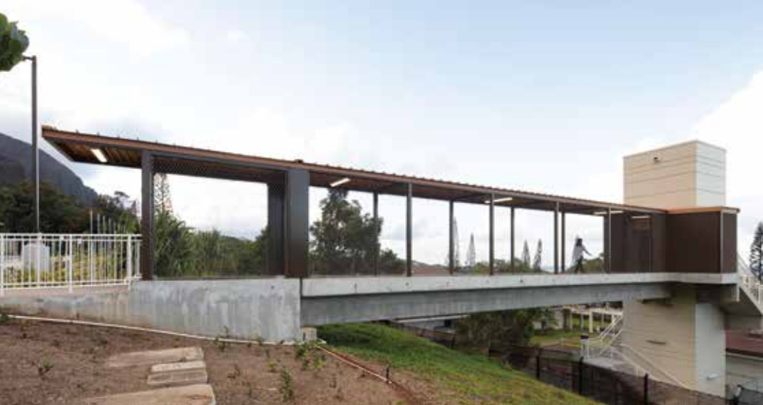
Figure 4. Double tee bridge with site elevator/stair tower.
