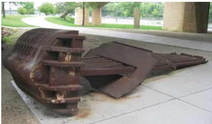
A portion of the cast iron anchor blocks and wrought iron anchor chains on display at a nearby park – eight in total, two at each end of the cable.
