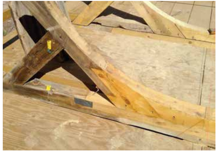
Figure 3. A typical repair of a bent by splicing new timber.
