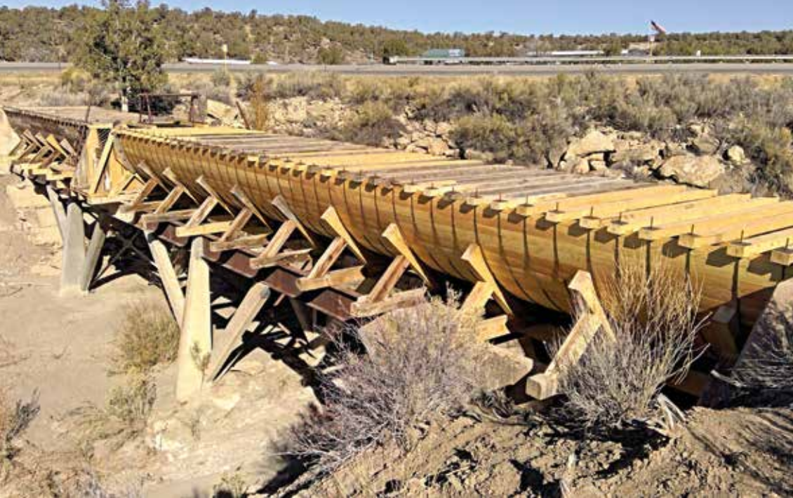
Figure 4. The McElmo Flume after rehabilitation.
