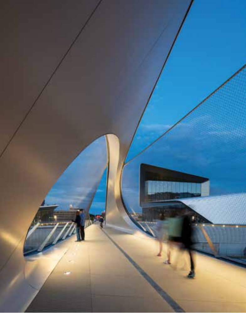
Figure 4. Inside view showing translucency of parapets required over rail tracks. Courtesy of Jason O'Rear.
