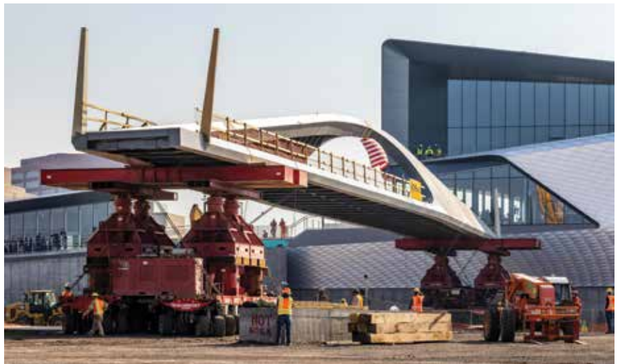
Figure 5. Bridge erection using SPMTs.
