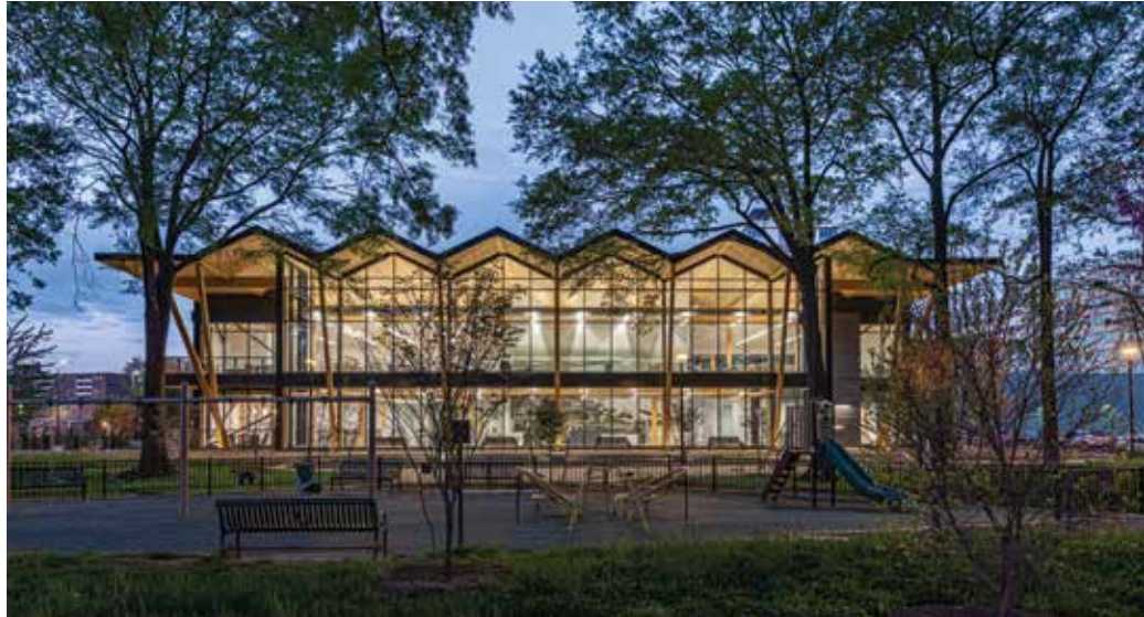
StructureCraft was an Outstanding Award Winner for the DC Southwest Library Project in the 2021 Annual NCSEA Excellence in Structural Engineering Awards Program in the Category – New Buildings under $30M.
