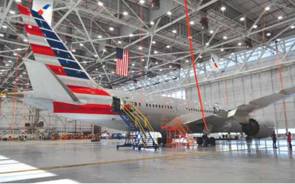
American Airlines Hangar 2 at O'Hare International Airport in Chicago, IL, was completed 14 weeks early due to incorporating construction engineering and detailing early on in the project.
