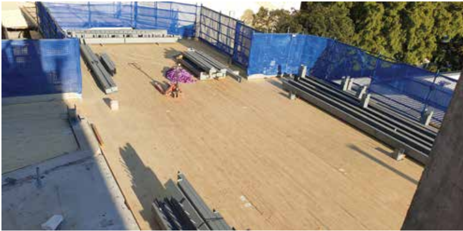
Level 03 under construction.
