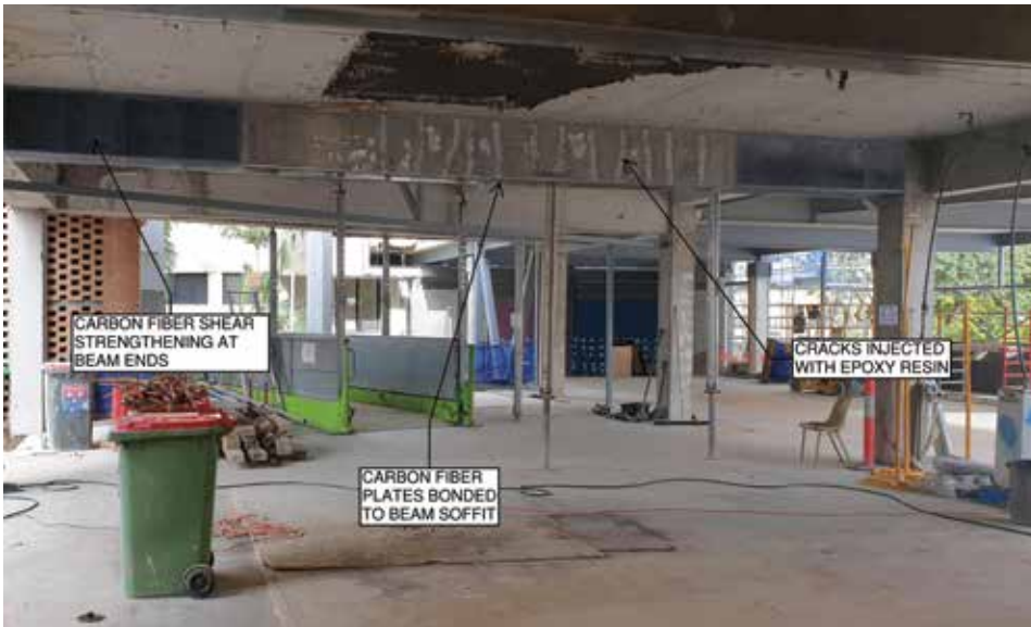
Carbon fiber strengthening to level 03 RC beams.
