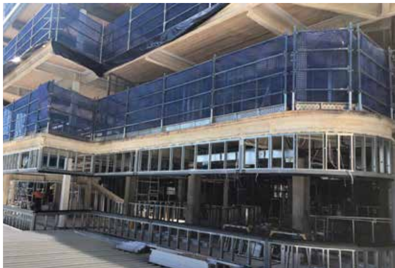
Southern elevation prior to the installation of cladding and curtain wall.
