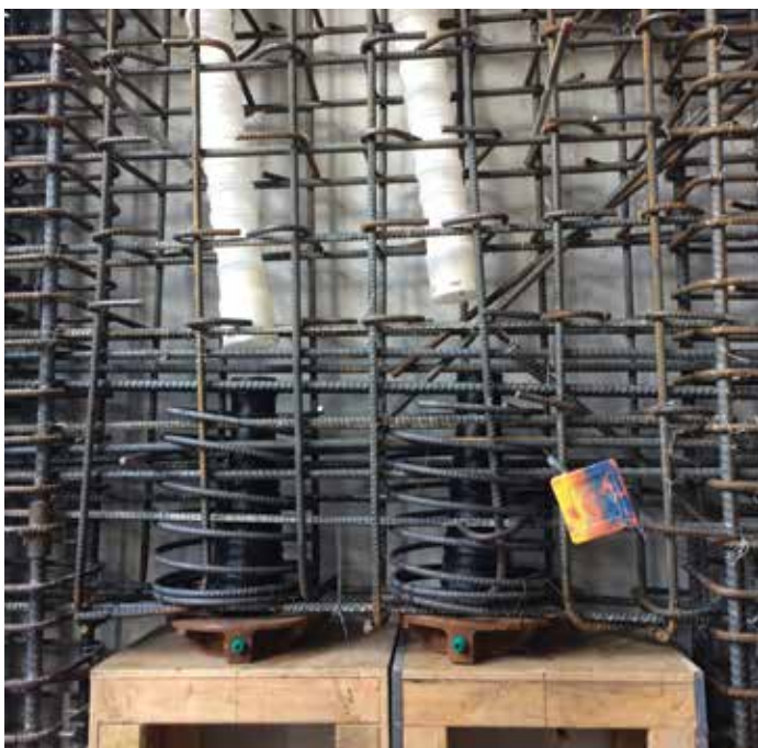
Post-tensioning anchorage and ducts.
