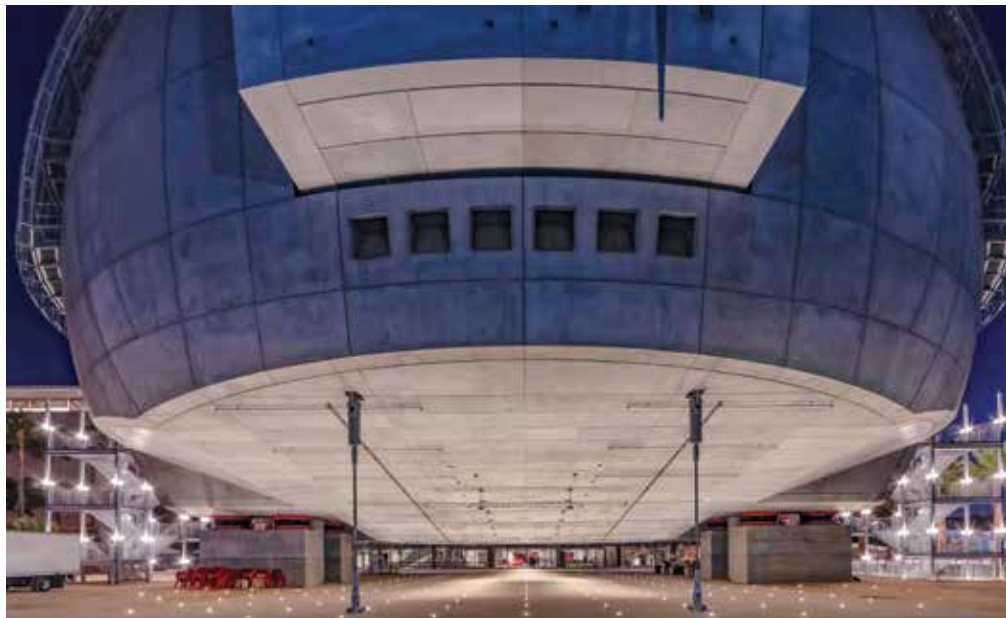
The theater volume is framed by spherical, reinforced concrete walls, capped by concrete slab-on-deck above a spider web grillage of steel beams, which effectively create a very shallow dome to complete the primary structure and provide support for the glass-enclosed terrace above. Courtesy of Gabe Guilliams, Buro Happold.
