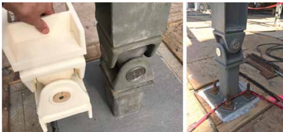
The finished column hinges were cast from high-grade carbon and stainless steel alloys, providing a streamlined construction and fabrication process and ensuring an aesthetically pleasing final product.
