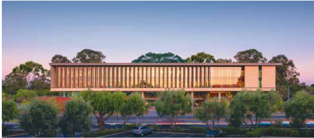
HOK was an Outstanding Award Winner for the Stanford Center for Academic Medicine Project in the 2021 Annual NCSEA Excellence in Structural Engineering Awards Program in the Category – New Buildings $80M to $200M.
