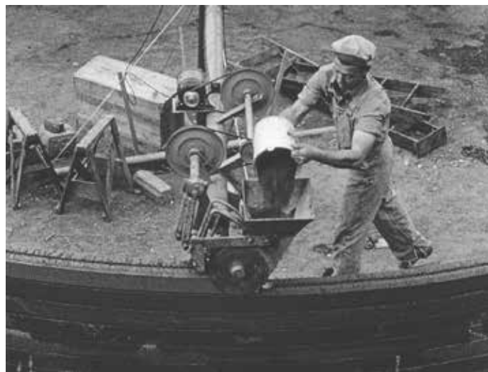
Figure 2. Molding elements were added to the extruder, creating interlocking channels between layers and emphasizing the distinct appearance of a printed structure. Courtesy of David Tippold – Urschel Laboratories, Inc.
