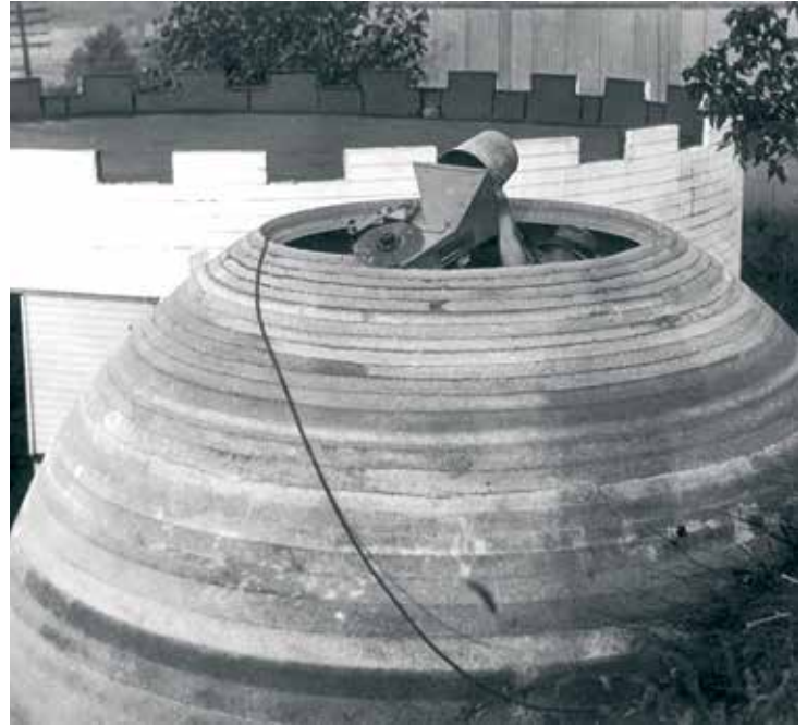
Figure 5. A domed structure is being constructed by one person and a Wall Building Machine, a feat yet to be accomplished with a modern printing system at this scale. Note the decreasing layer height as slope increases, a technique now used in modern 3-D printing systems to manage overhanging layers. Courtesy of David Tippold – Urschel Laboratories, Inc.
