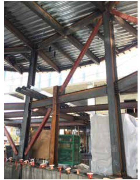
Braced frame at City Hall Council Chambers.
