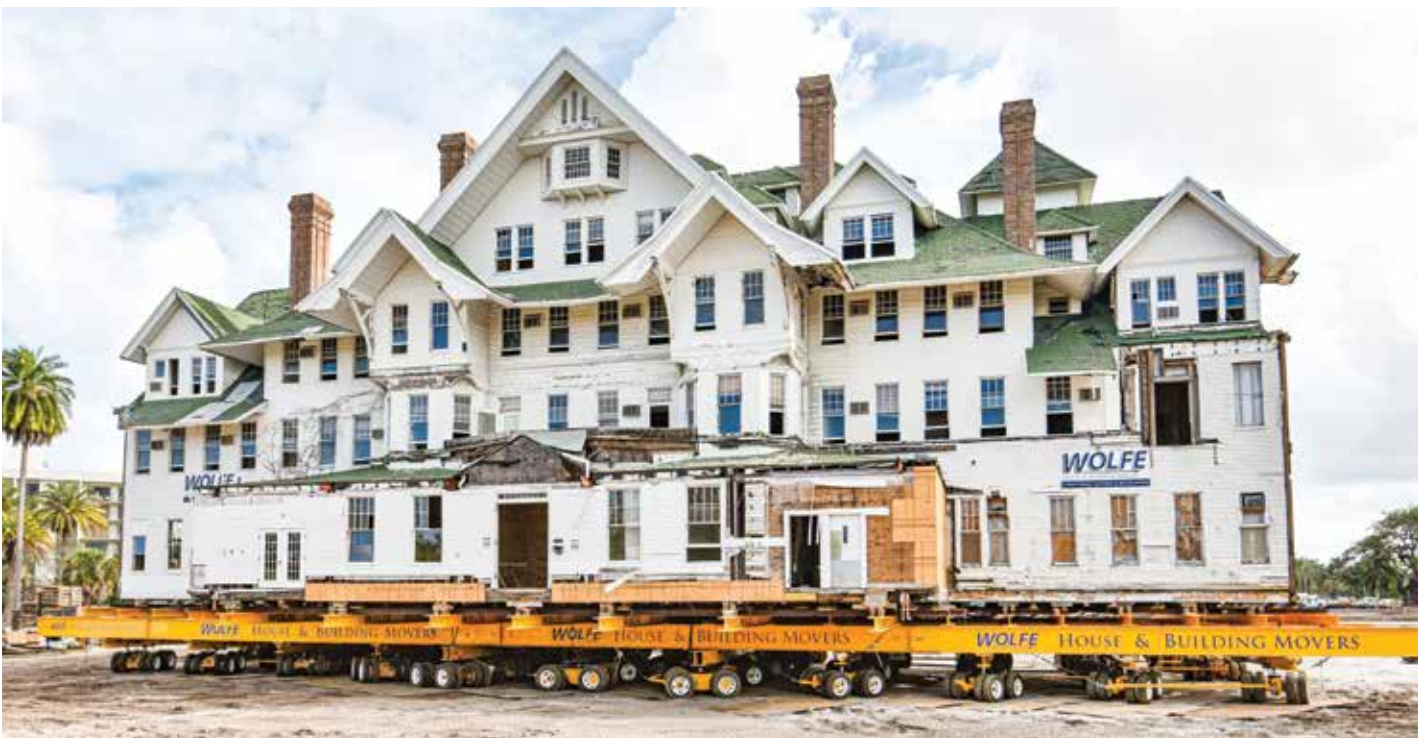
Moving of the Hotel. Courtesy of Wolfe House & Building Movers.
