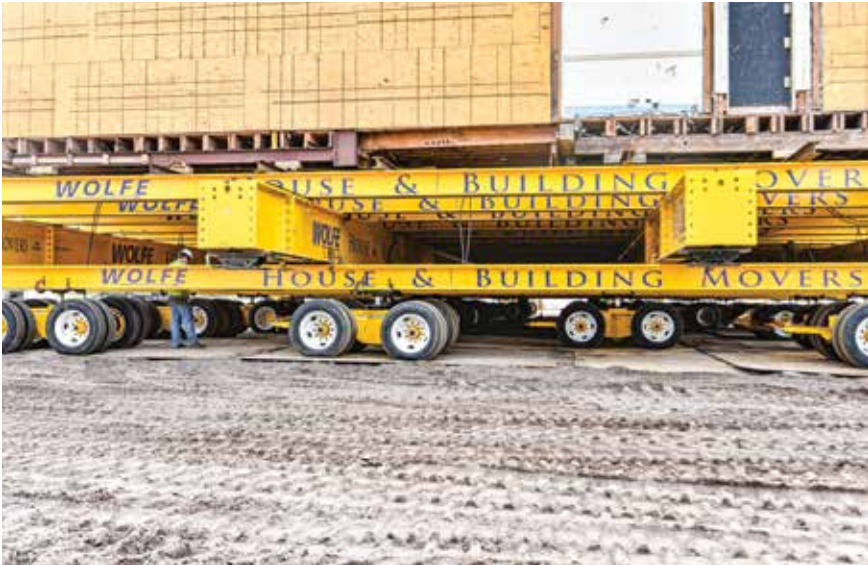
Wheeled dollies. Courtesy of Wolfe House & Building Movers.
