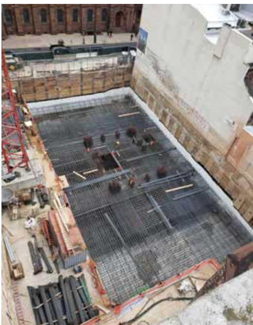
Mat foundation reinforcing steel.
