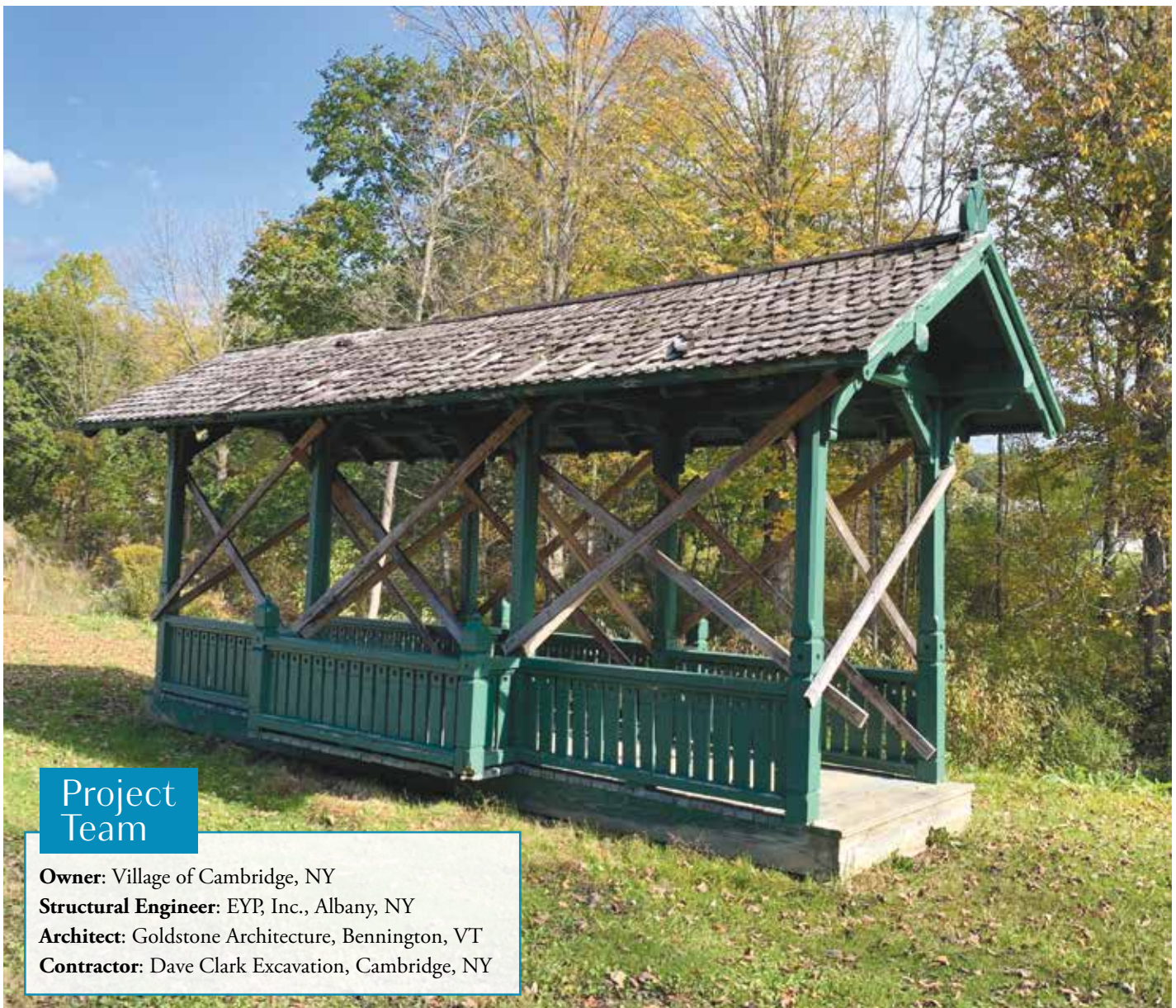
Bridge in storage off-site at the Village DPW yard; note that many diagonal braces were added to stabilize the bridge during lifting and transportation.
