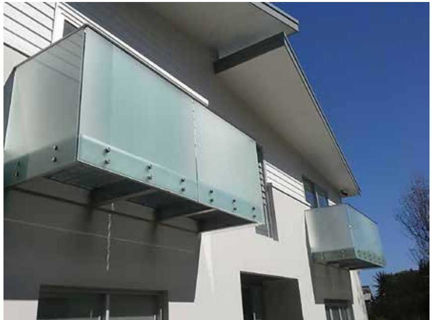
Figure 3. Point-Supported glass railing (Bing Image Free Use Search).
