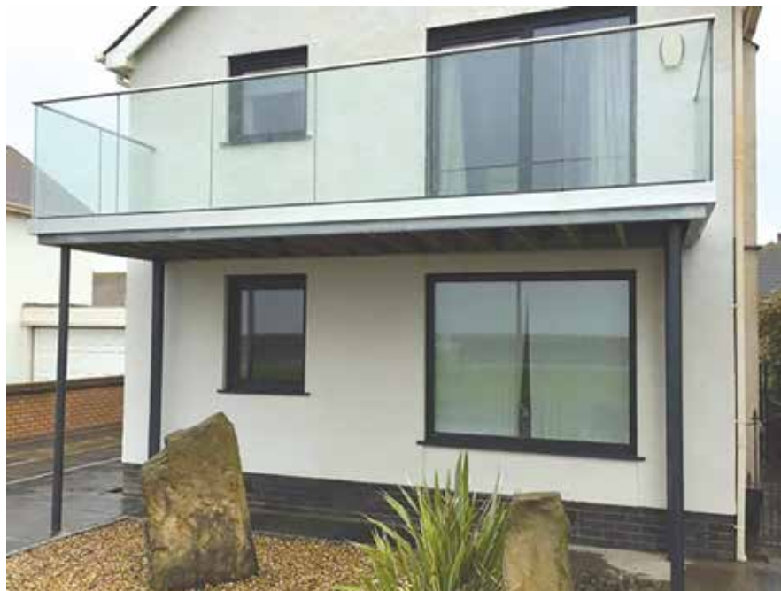
Figure 2. Base shoe glass railing (Bing Image Free Use Search).
