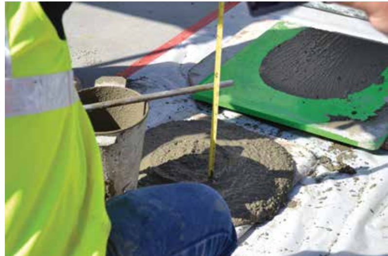
Grout must be high slump to allow flow in masonry cells.
