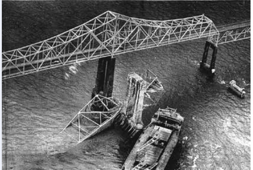
Ship and bridge after the collapse; rammed pier center-right.
