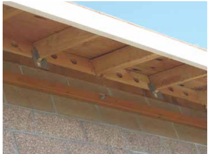
Anchor bolts are used to attach the wood ledger to the side of the masonry wall.
