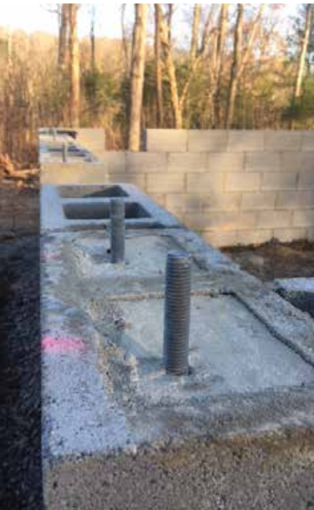
Anchor bolts at the top of wall. Courtesy of the Southeast Concrete Masonry Association
