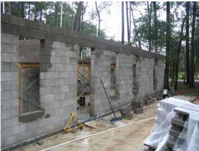
Figure 5. Residence in Texas (wall construction and before stucco application). Courtesy of Cercorp Initiatives Inc. ( www.cercorp.com ).
