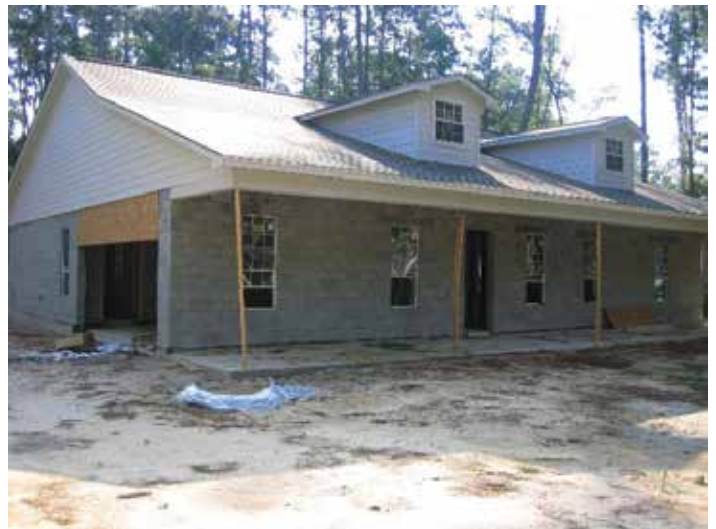
Figure 5. Residence in Texas (wall construction and before stucco application). Courtesy of Cercorp Initiatives Inc. ( www.cercorp.com ).
