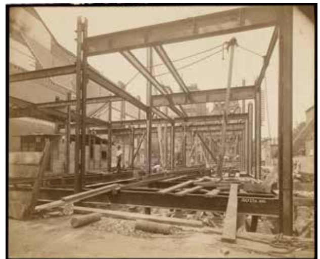
Figure 25. Ongoing erection of the first and second-floor framing.
