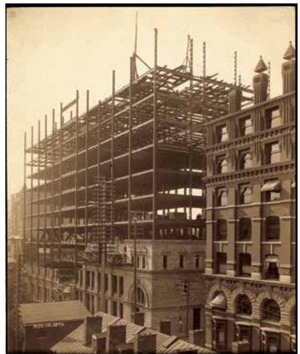
Figure 28. Partially erected tower and lower façade.
