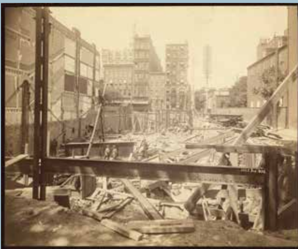
Figure 24. Initial erection of the first-floor framing.
