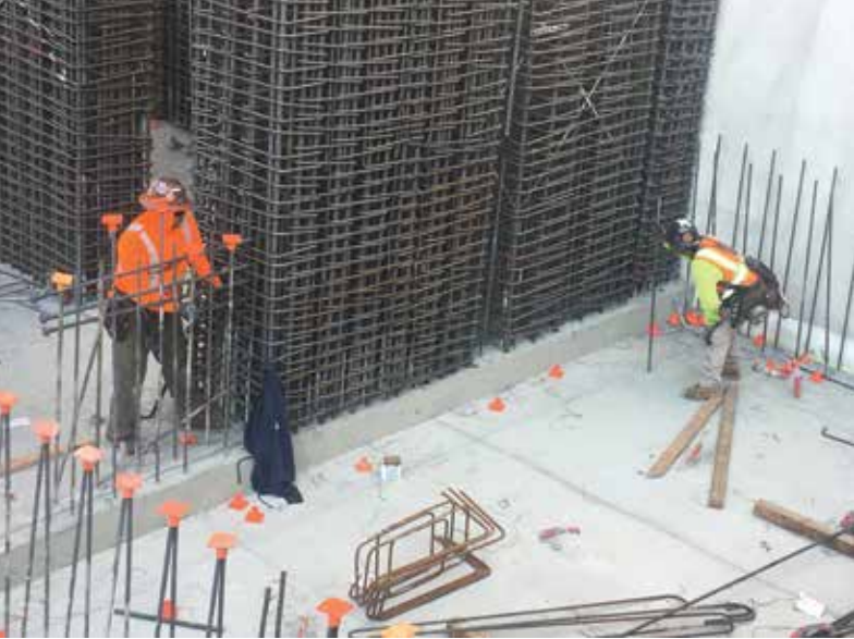
Inspection of shear wall reinforcing.
