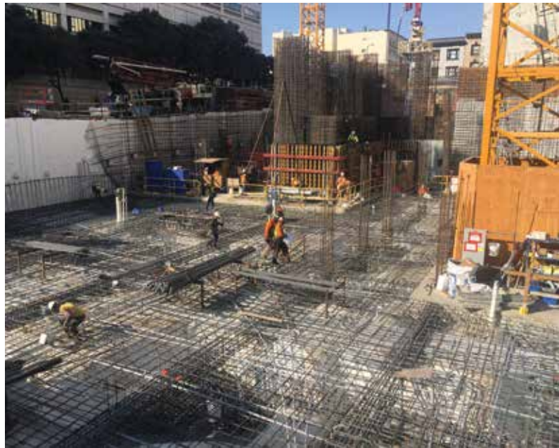
Inspection of concrete flat work.
