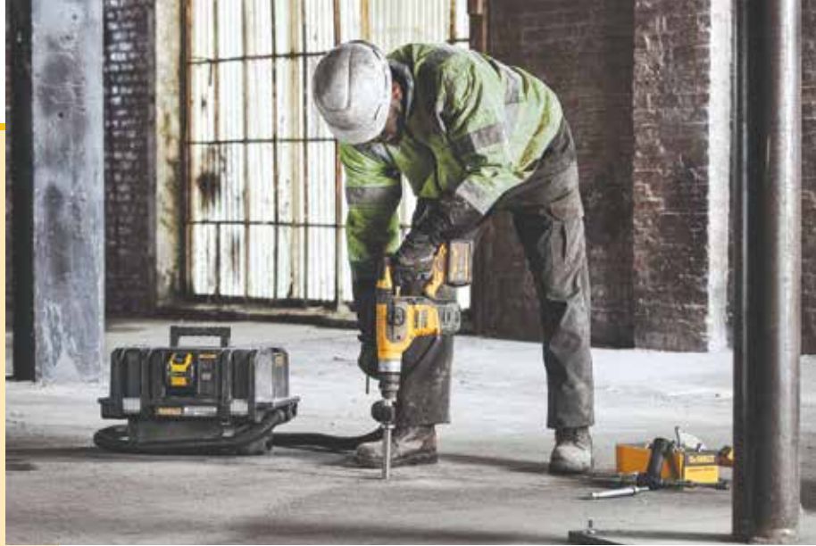
Figure 3. The complete undercut anchor system: anchor, primary drill bit, undercut bit, setting tool, hammer drill, dust extractor.
