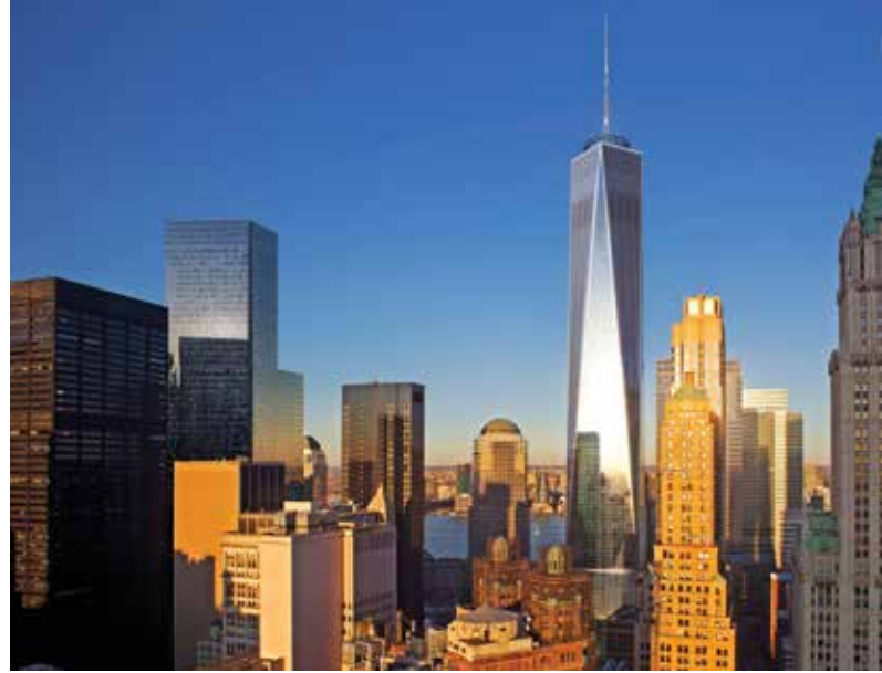
The high-strength concrete used in the One World Trade Center was designed with fly ash, silica fume, and slag cement SCMs.
