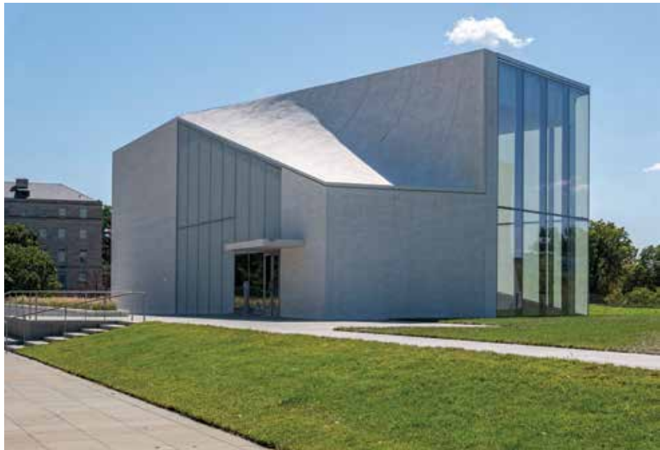
The conical slab comprises a gray structural concrete layer, a roofing membrane, and a white exterior layer. The form was achieved using both formed concrete and shotcrete placements.
